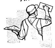
Drying time between ground coat and finish coat — several days with ordinary plasters—reportedly can be cut to one day by use of a plaster composed of zinc stearate, ground marble aggregate, hydrated lime, cement and color.
